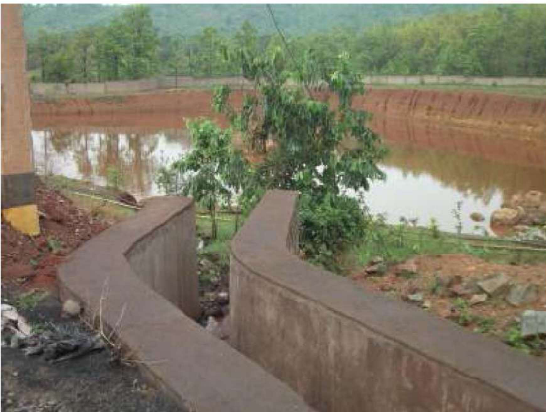
Fig. 5.7: Part of Implemented Drainage Network Connecting Reservoir
