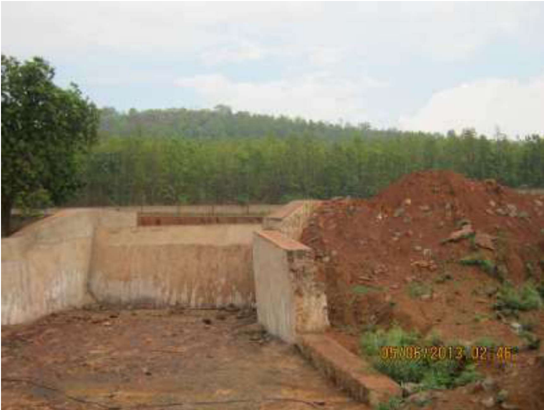
Fig. 5.6: Implemented Check Dam
