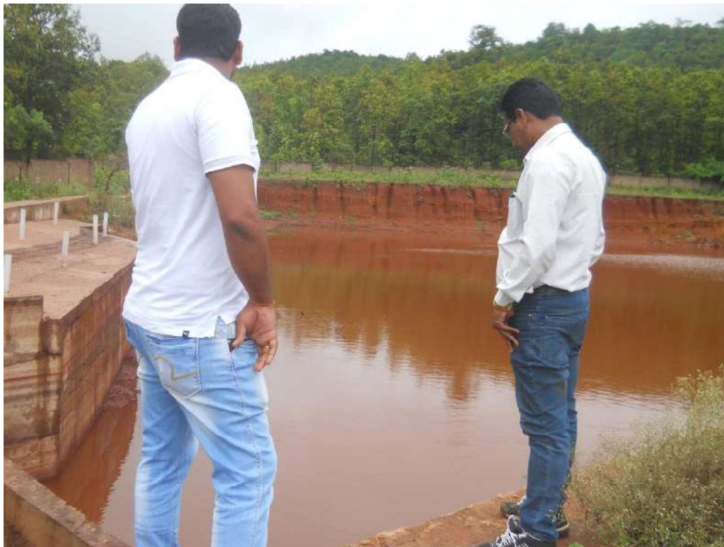
Fig. 5.5: Existing Rain Water Harvesting Reservoir with Check Dam
