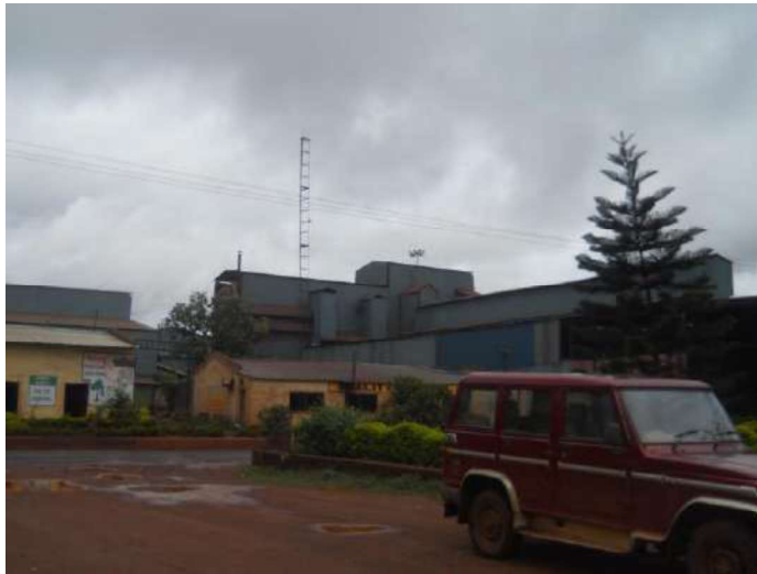
Fig. 5.8: Photograph showing Roof Top Clusters for Proposed Rain Water Harvesting & Artificial Recharge
